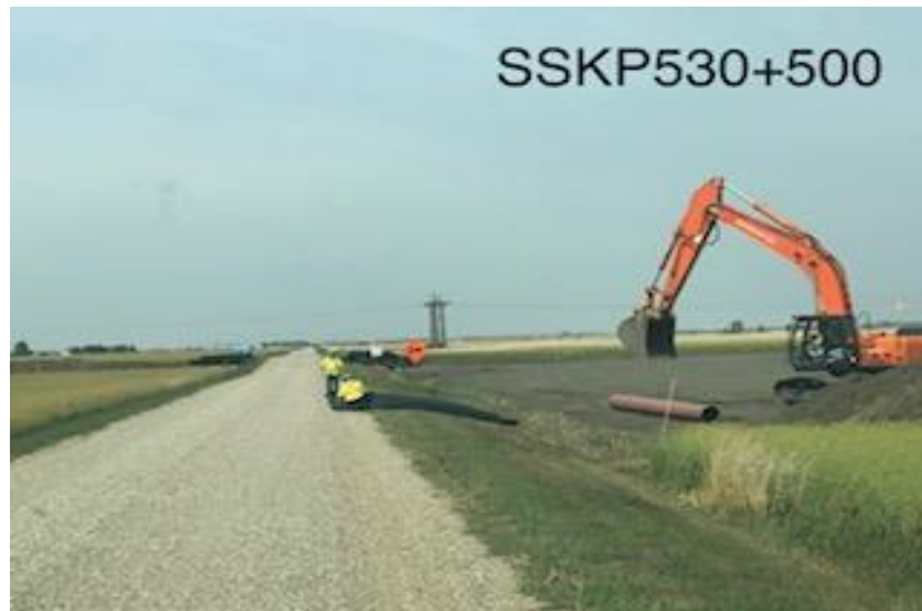
Ramp installation, geo tech being used
