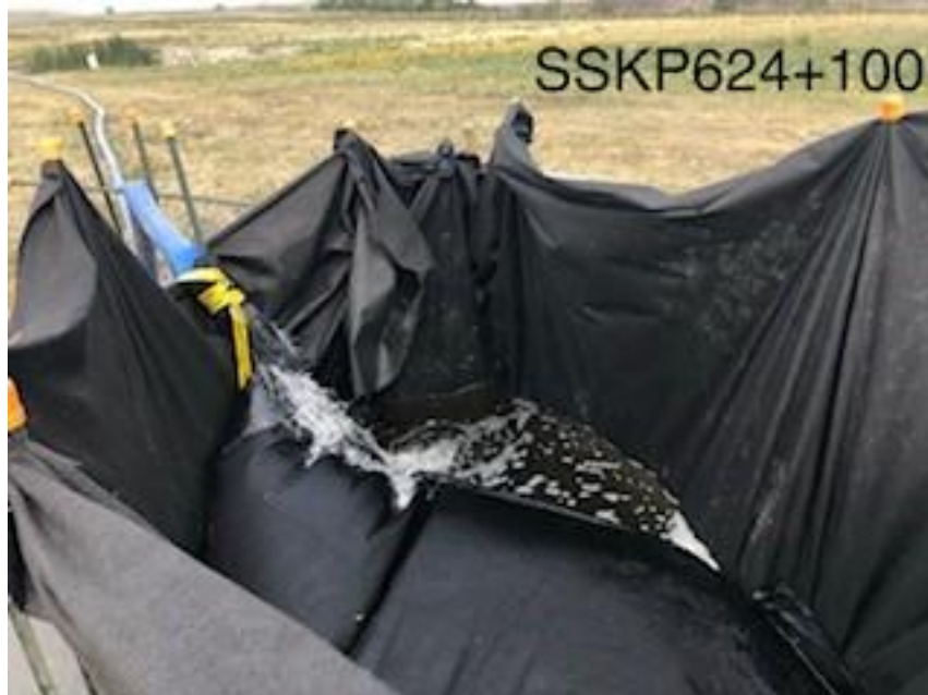
Banister crew set up an area near a dug out being pump out
