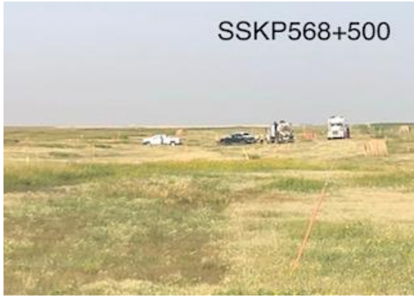
Hydro Vac trucks day lighting underground lines “Hot lines”
