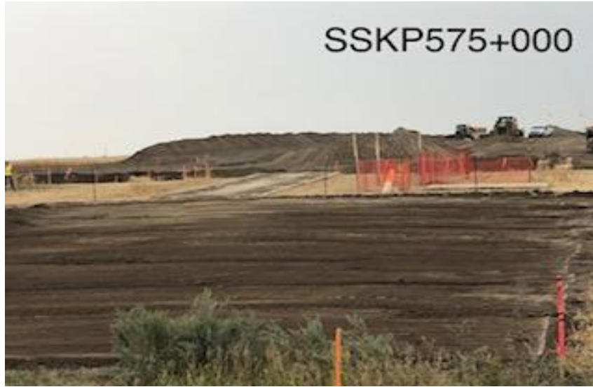
Ramp installation over hot lines
