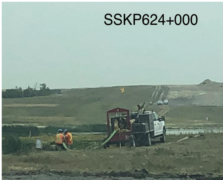
Banister crews prepping to drain a body of water
